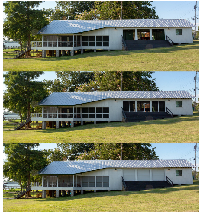
Figure 5. Open/screened/closed openings. Image credit Jim Osborne.
